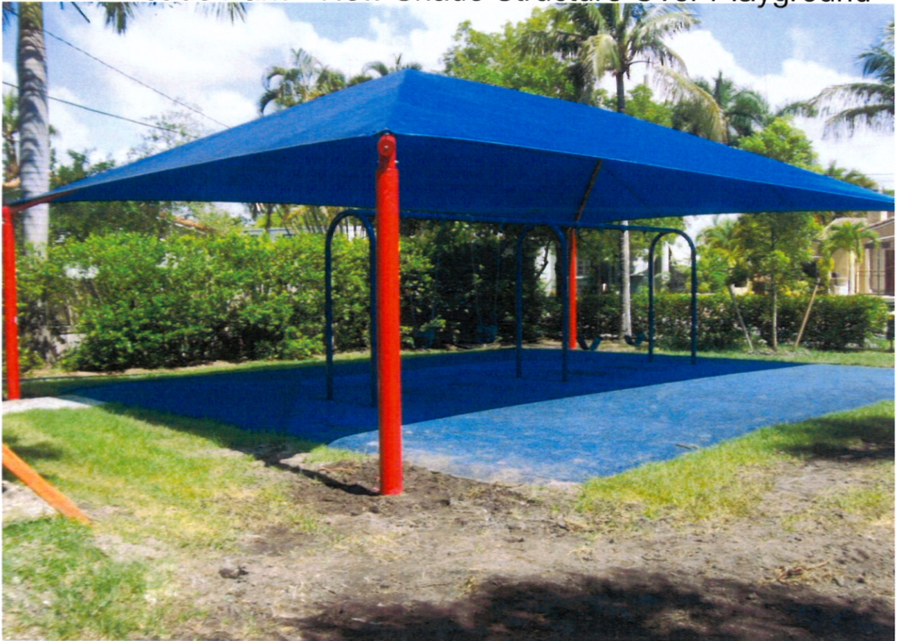
Belle Meade Park - New Shade Structure Over Playground
