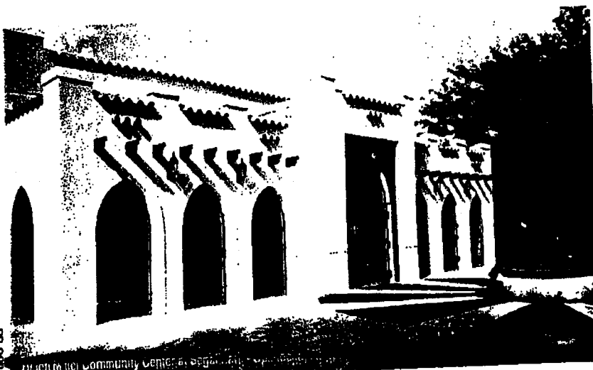
Recreation Community Center - Spring Hill, Florida
