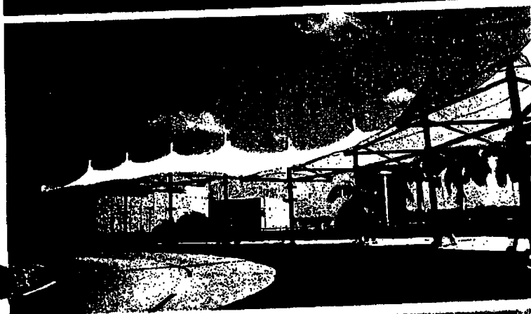
Broward County Curbside Pedestrian GTA Canopies
