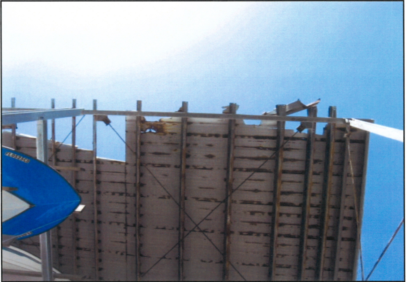
MARINE STADIUM MARINA BOAT RACK METAL ROOF DECK REPLACEMENT
