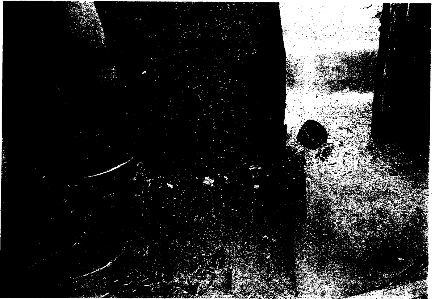
Completely exposed column showing corrosion
