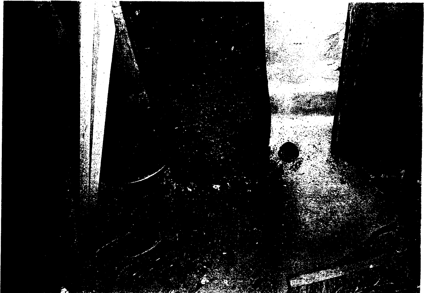
Completely exposed column showing corrosion
