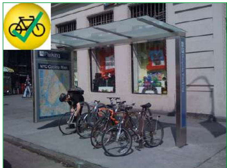
Figure 7- 12: Conveniently Located Bicycle Parking Shelter
