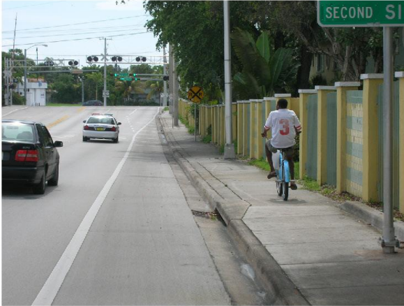
NE 54 Street is designed so that most bicyclists opt to use the sidewalk.
