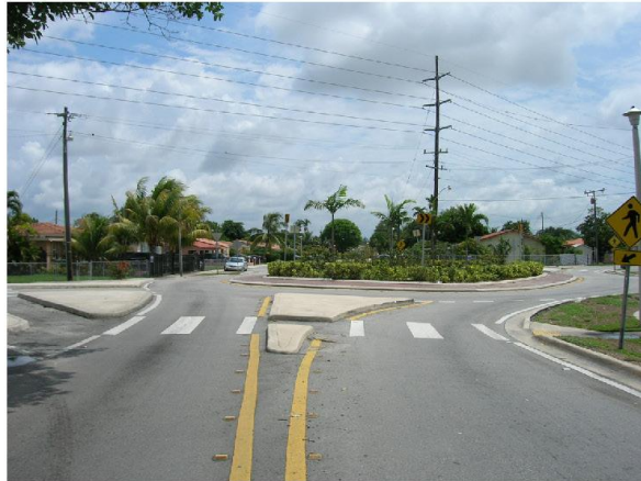
A traffic circle at SW 4th Street and Tamiami Boulevard improves safety.
