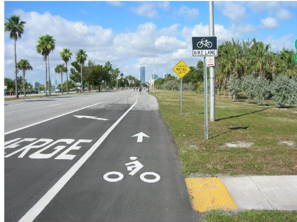
Recent improvements have made the Rickebacker Causeway safer.
