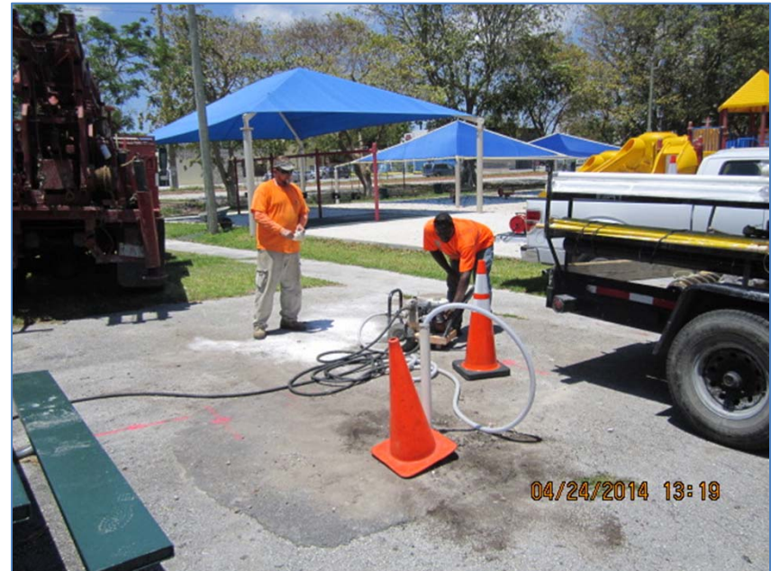
Monitoring well development activities at MW-2
