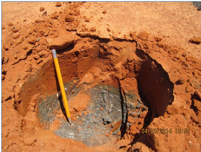
At SB-22, the infield clay/sand mix was only 4" thick followed by incinerator ash fill material
