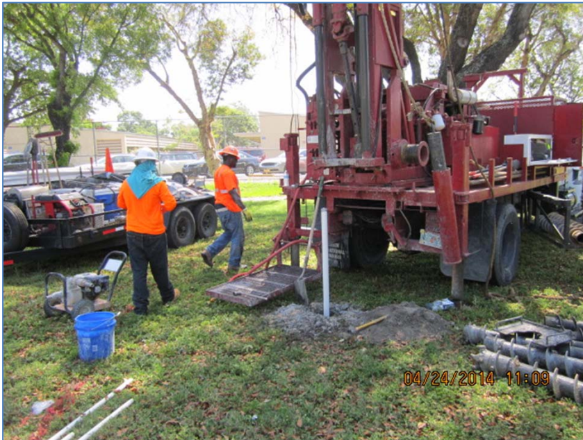
Monitoring well installation activities at MW-1
