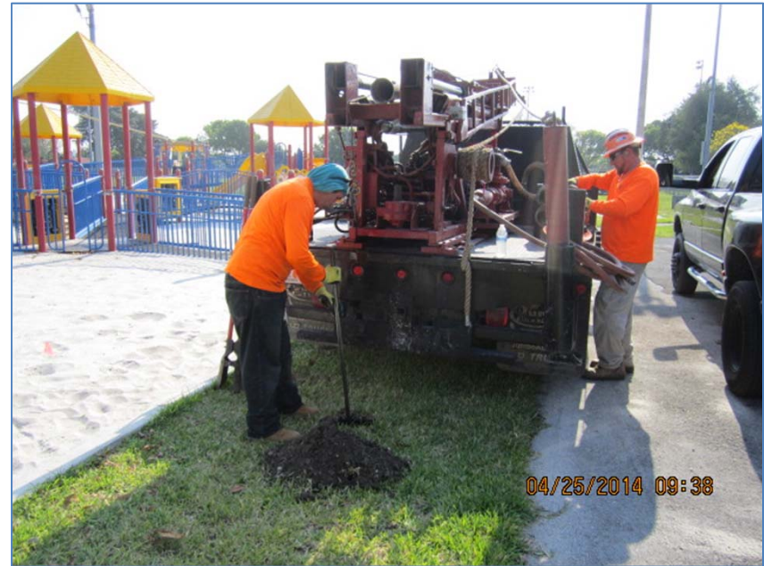
Methane gas probe installation activities at MP-4
