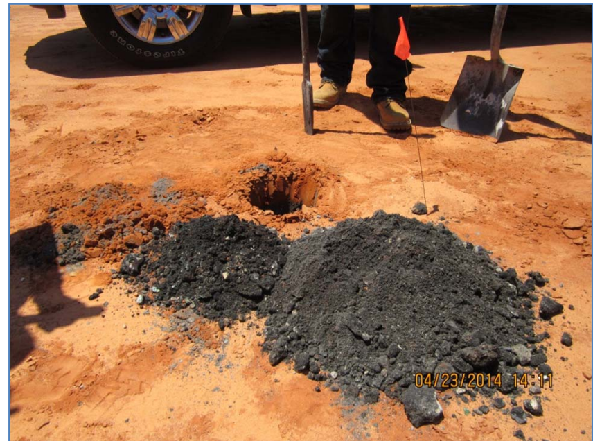
Incinerator "ash fill" material and stained residues in the infield at SB-22
