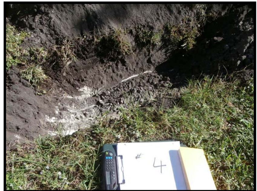
Test Pit 4. No debris.
