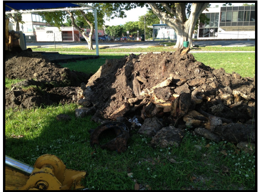
Test Pit 12. C+D debris.
