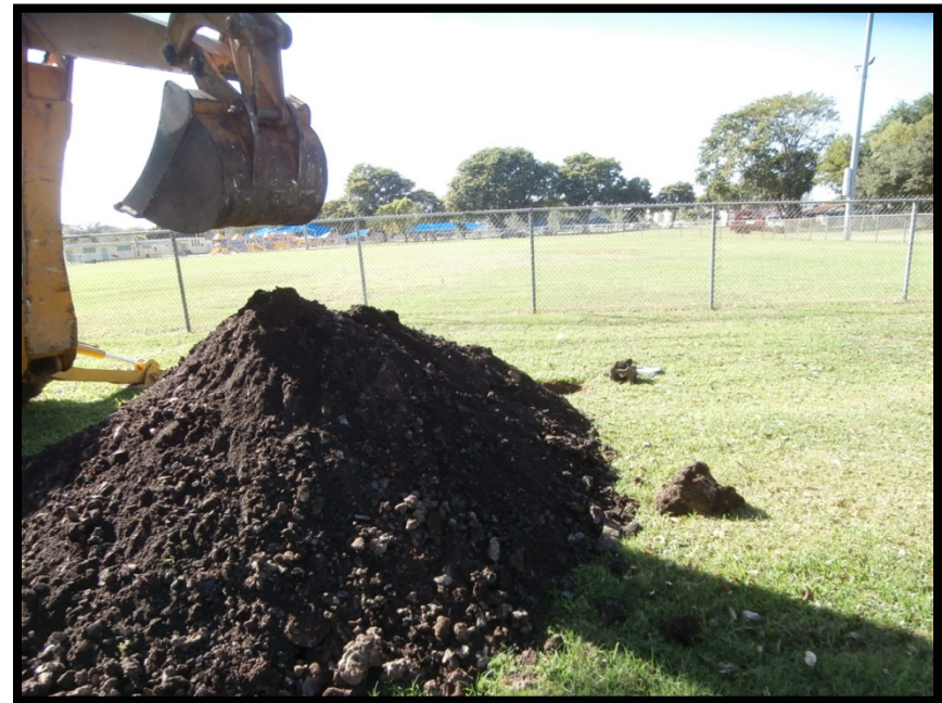
Test Pit 8. Dark colored soil mixed with limerock.
