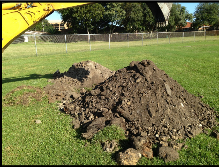
Test Pit 13. C+D debris
