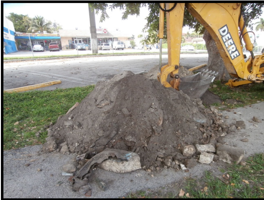
Test Pit 3. Bottles, rubber pieces and C+D debris.
