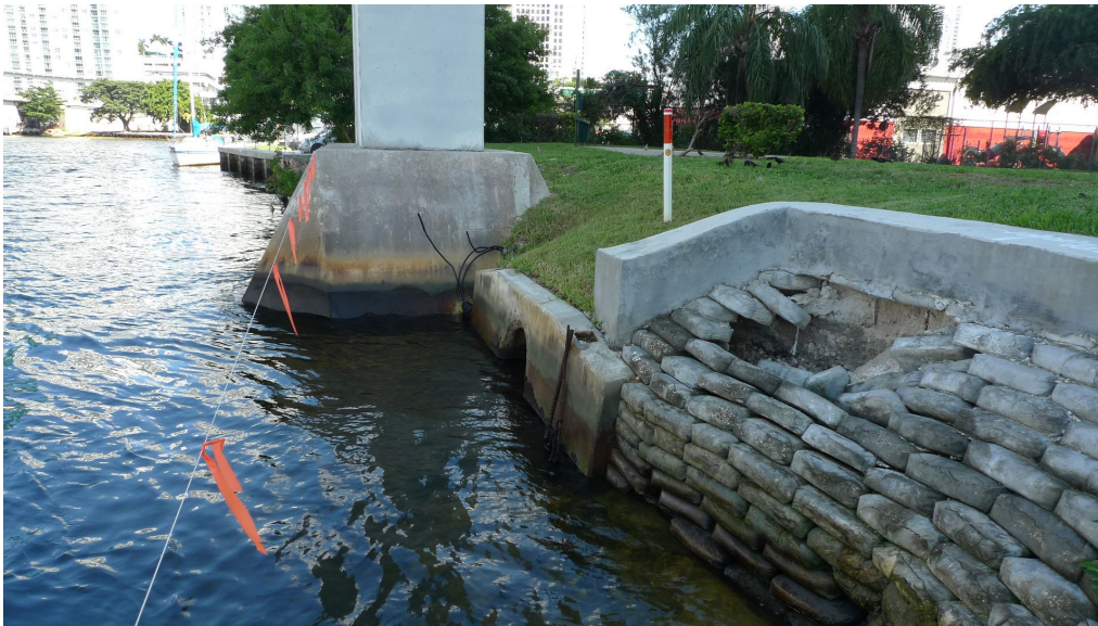
FIGURE 12 CURRENT STATE OF SW 1 ST COURT OUTFALL
