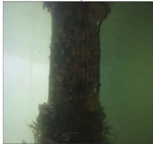
Pier 3 PC12E Top Below Water
