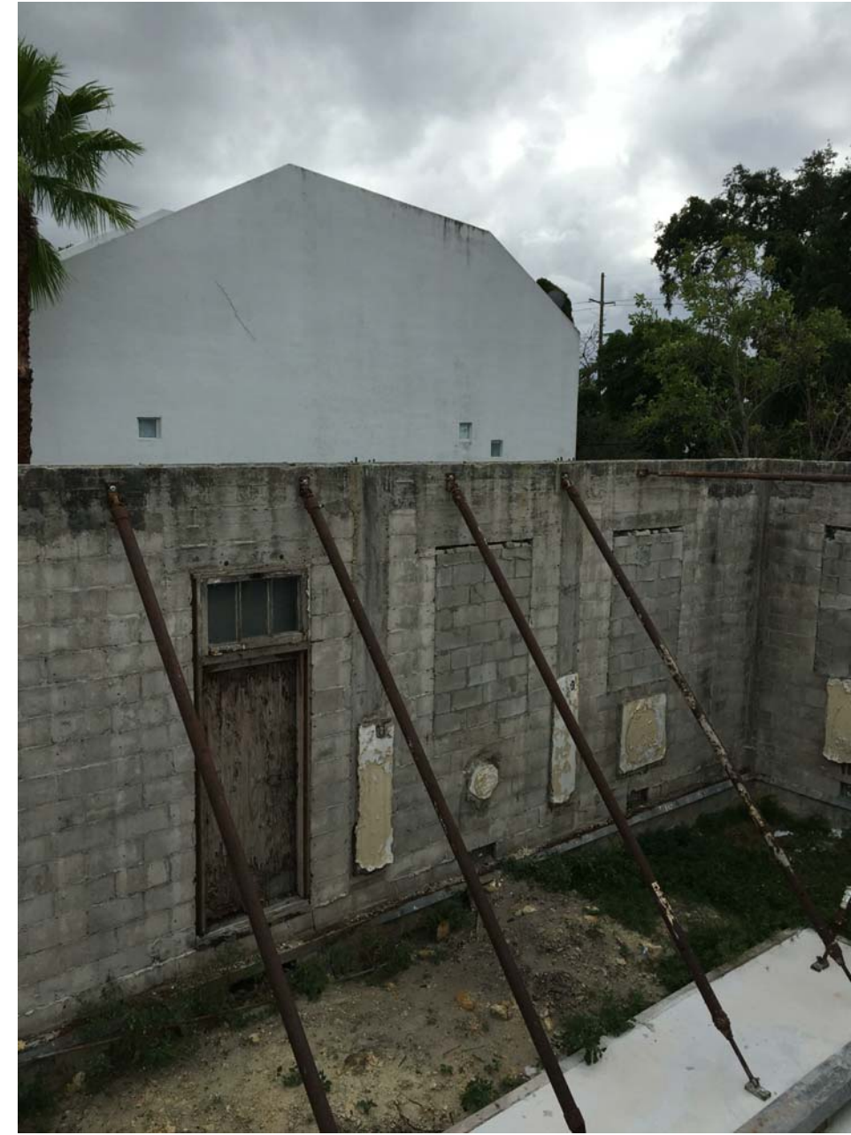
VIEW OF EXTERIOR SOUTH WALL SHORING SEEN FROM INTERIOR
