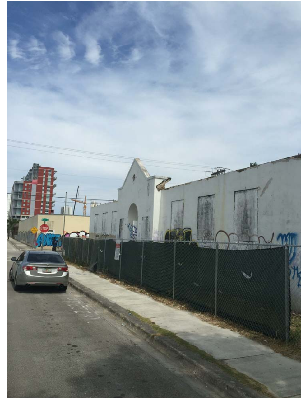
VIEW OF EXTERIOR BUILDING ALONG 17 STREET
