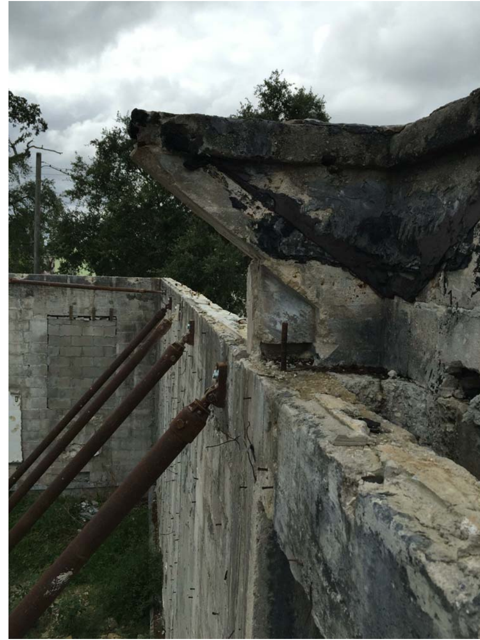
CLOSE UP VIEW OF SHORING AT TOP OF WALLS
