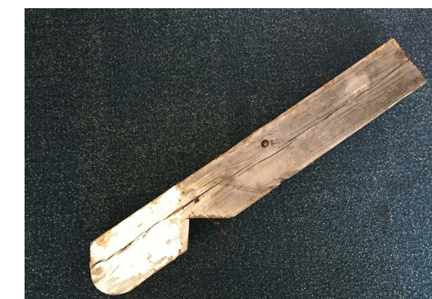
EXISTING INTERIOR CONDITION. WOOD FRAMING TO BE SALVAGED, REMILLED AND REPURPOSED IN RESTORATION
