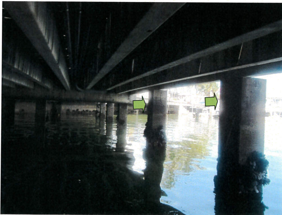
Photo 26: Free standing concrete piles under concrete joists.
