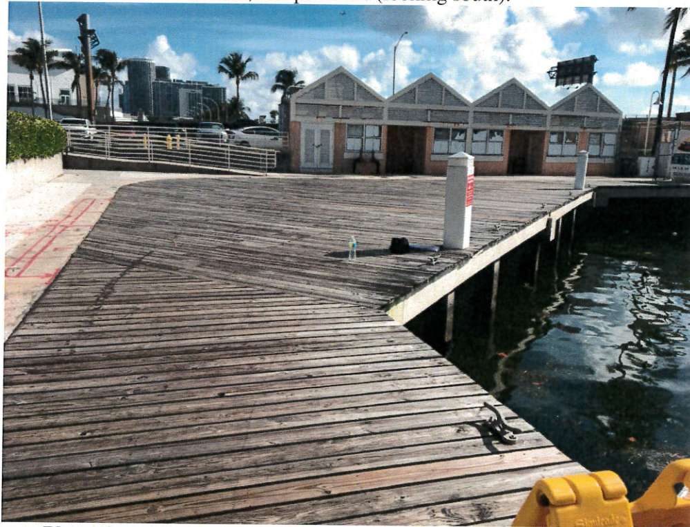
Photo 4: Existing wood deck corner, and pedestals (looking northeast).
