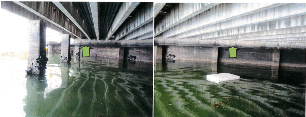
Photo 28: Southwest beam beyond (left photo), west beam abut to bulkhead through entire northwest corner of boardwalk (right photo).
