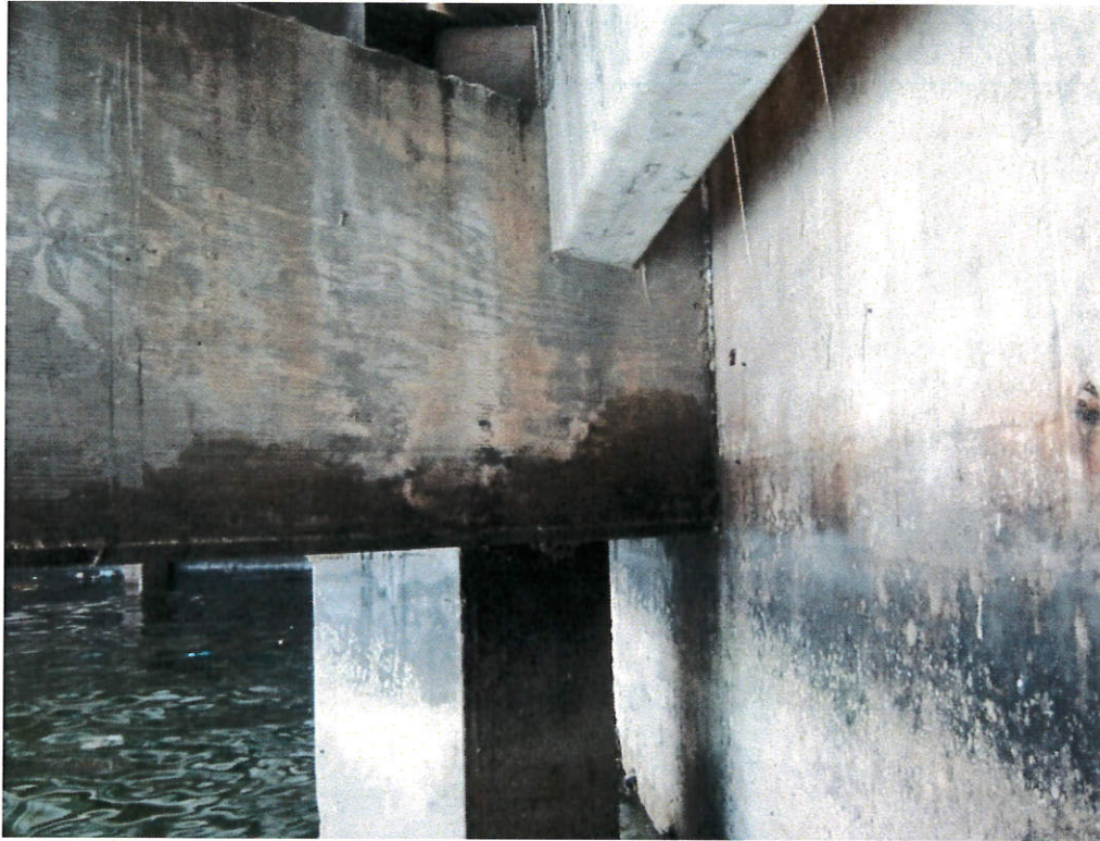
Photo 29: End of north beam abut to bulkhead.
