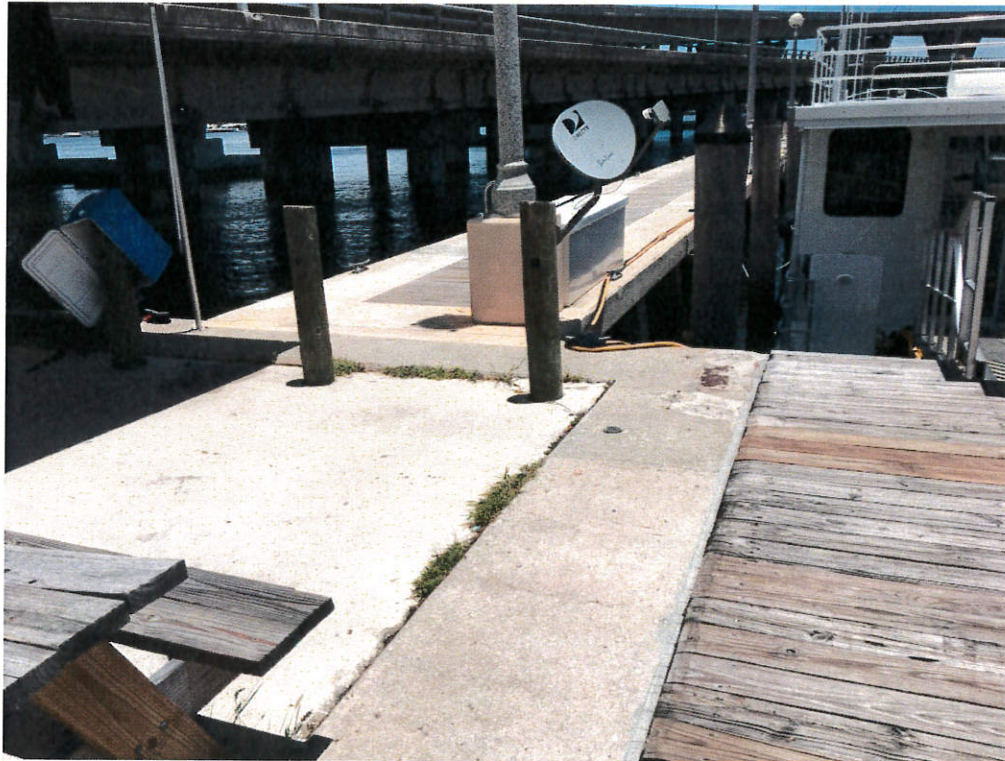
Photo 12: Transition from Pier 5 to Pier G (beyond).
