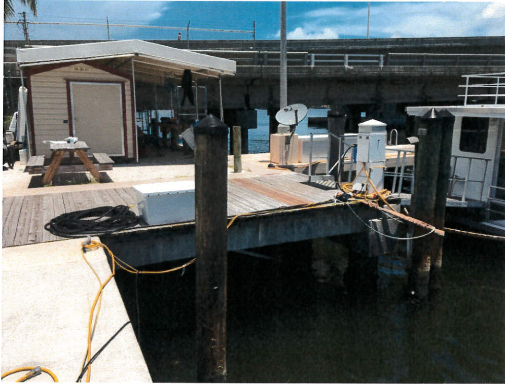
Photo 11: Transition from Pier 5 to Pier G (beyond).
