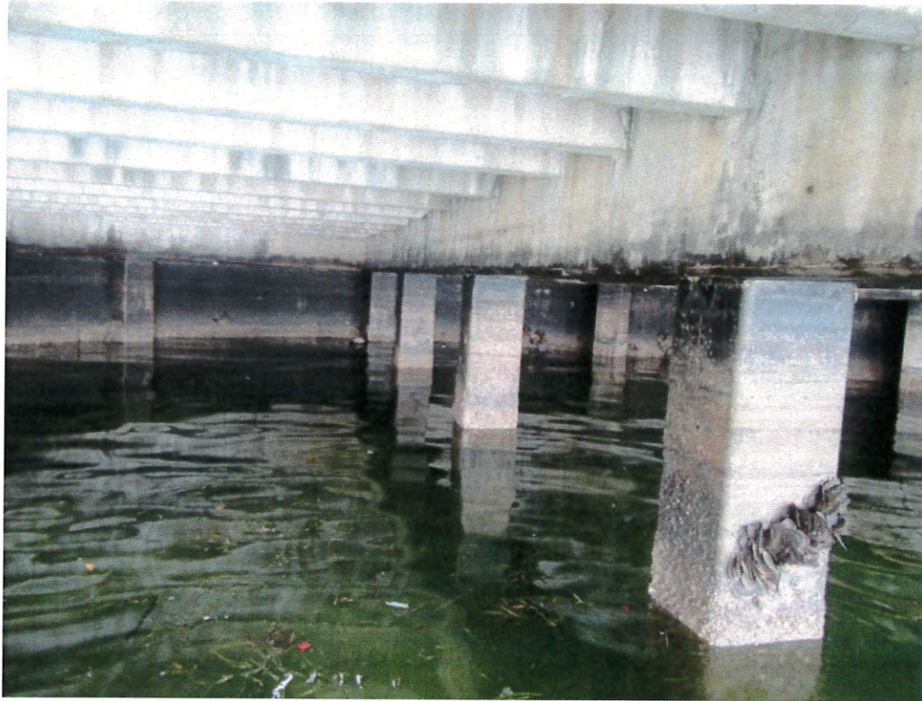
Photo 27: Center beam and piling (looking into northwest corner of boardwalk).
