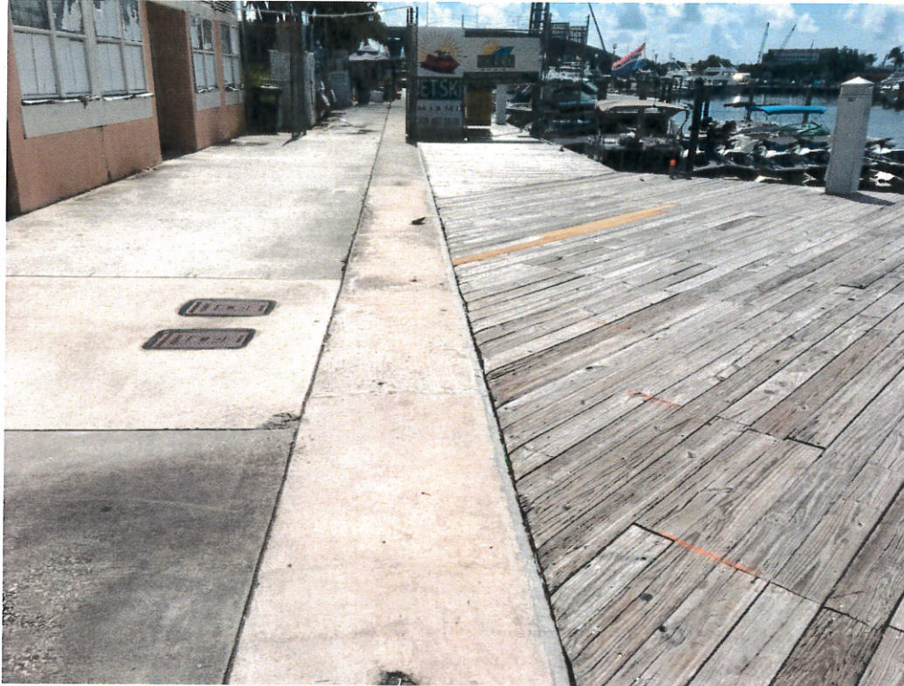
Photo 5: Existing bulkhead, sidewalk and wood deck (looking east).
