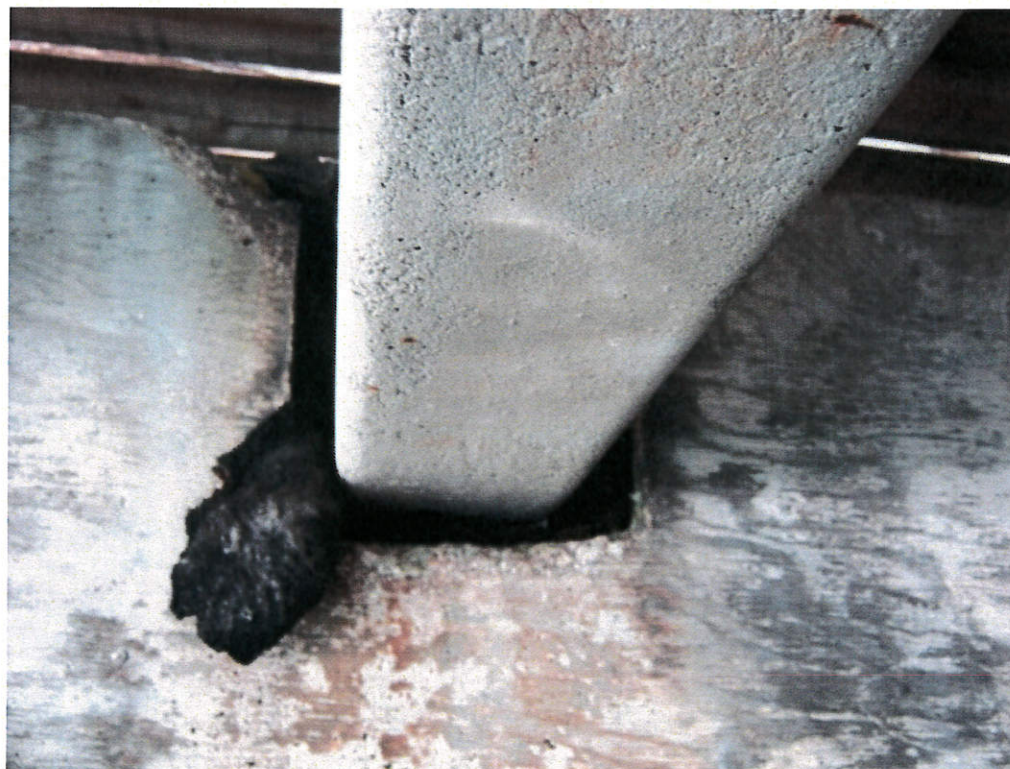
Photo 34: Existing concrete joists recessed into pile cap.
