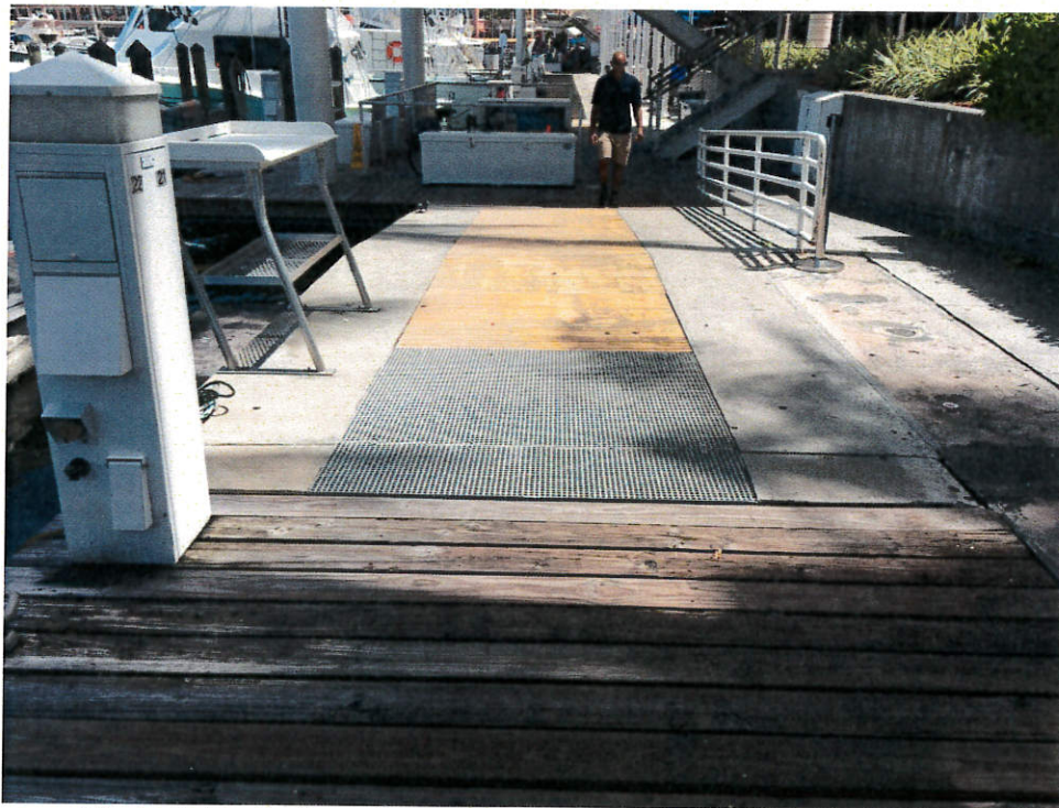
Photo 2: Beginning of wood decking construction (looking south).
