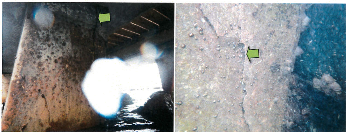
Photo 47: Pier G: couple of 18-inch x 18-inch piles exhibited up to 1/4-inch cracks.
