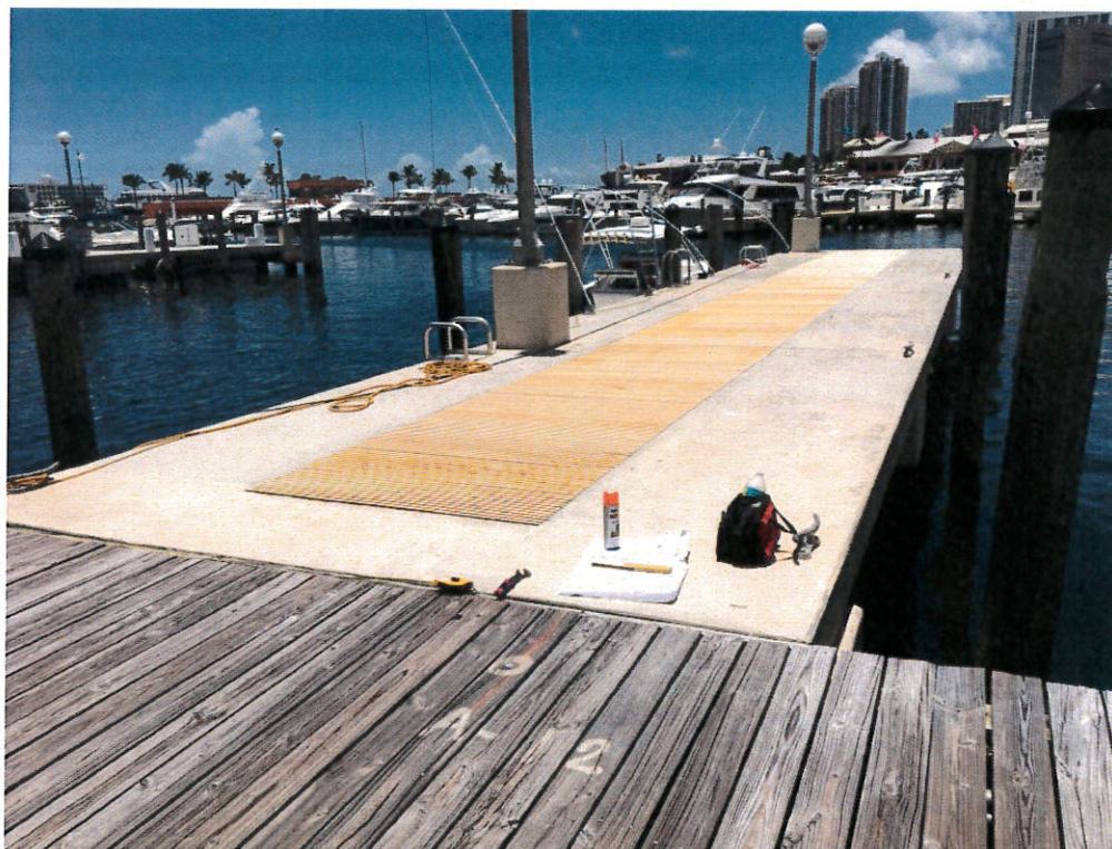
Photo 10: Existing Miami Fire Rescue concrete pier (looking southeast).
