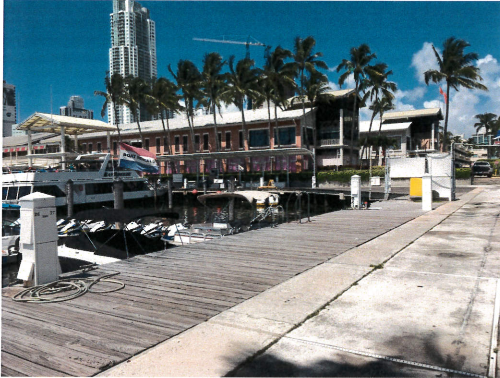
Photo 7: Existing bulkhead, pedestals, sidewalk and wood deck (looking west).
