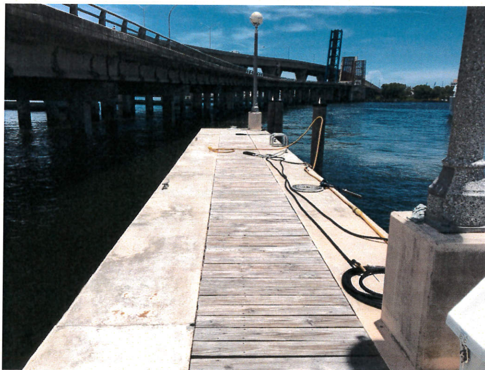
Photo 14: Existing Pier G (most eastern side).
