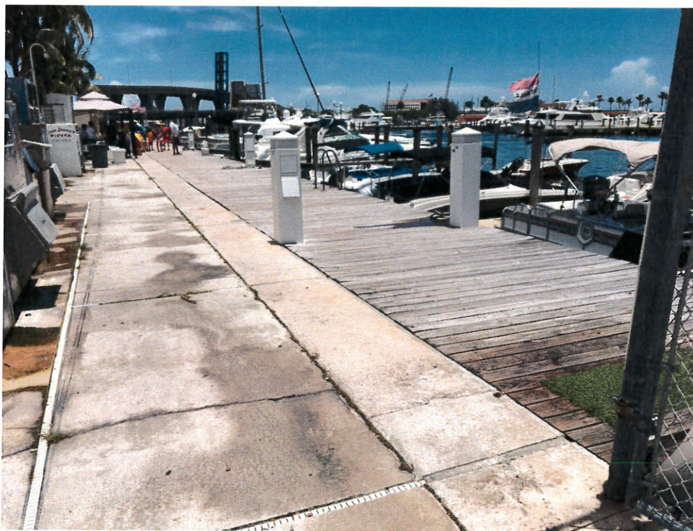
Photo 6: Existing bulkhead, pedestals, sidewalk and wood deck (looking east).
