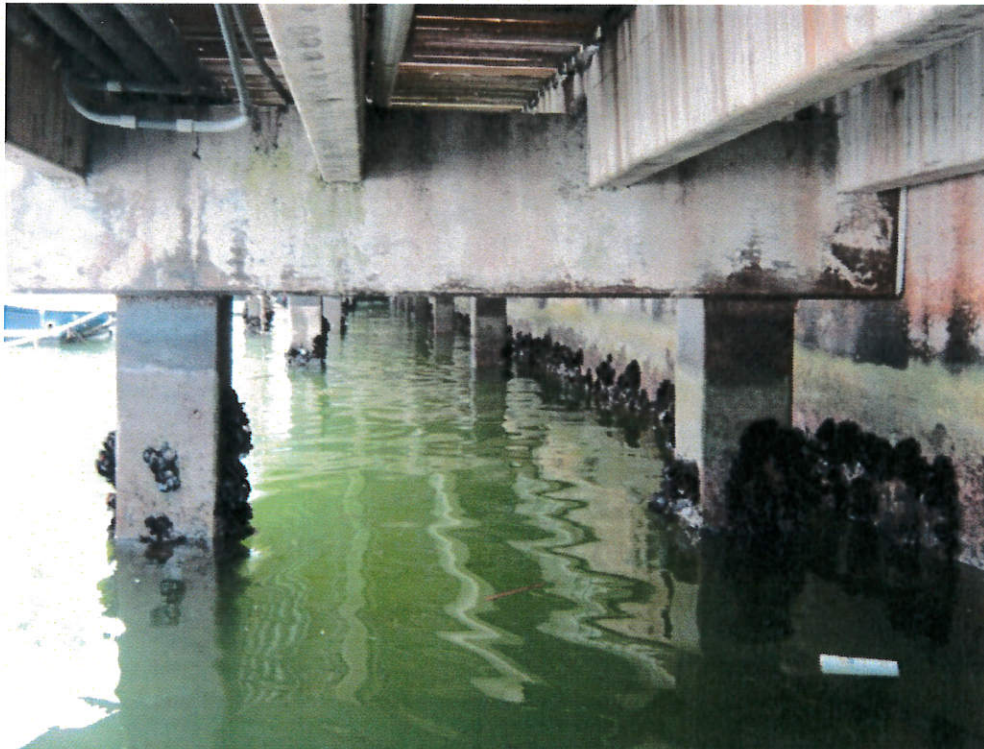
Photo 36: North segment of bulkhead exhibited more marine growth than the rest of wall.
