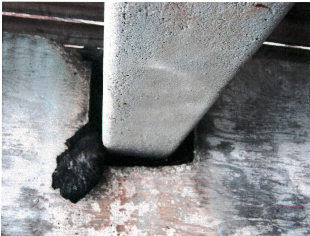
Photo 34: Existing concrete joists recessed into pile cap.
