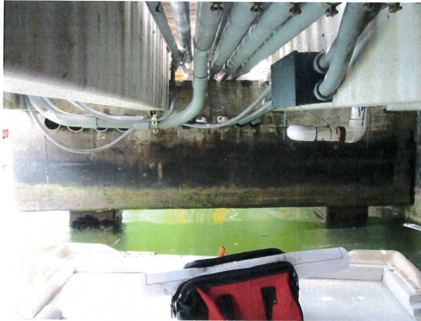
Photo 17: Underside at end of existing construction (wood decking and pre-cast concrete joists); this face of pile cap (Sta 0+00 looking south). Utility chase under wood decking from pile cap to pile cap.
