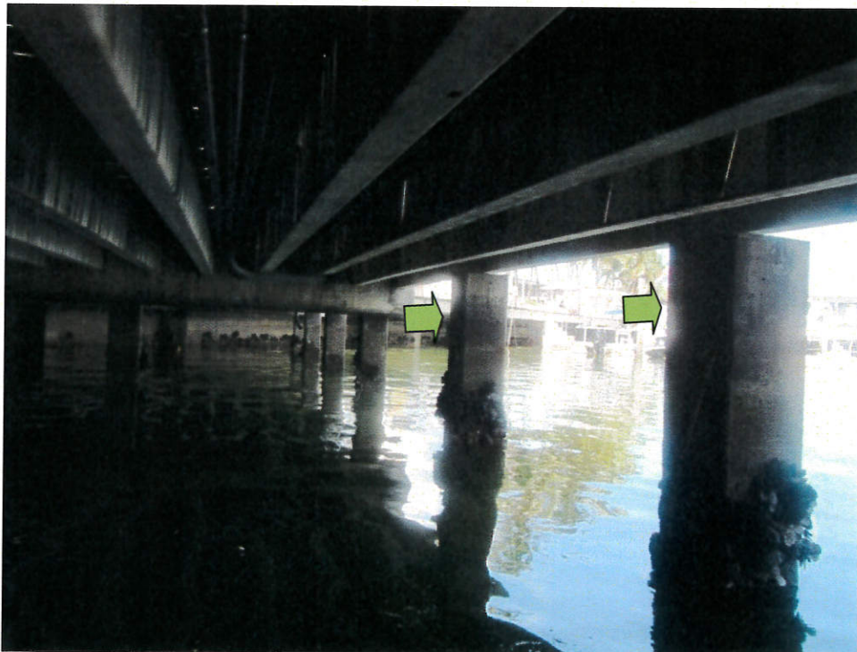
Photo 26: Free standing concrete piles under concrete joists.
