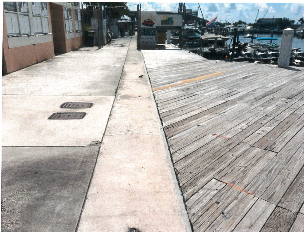
Photo 5: Existing bulkhead, sidewalk and wood deck (looking east).
