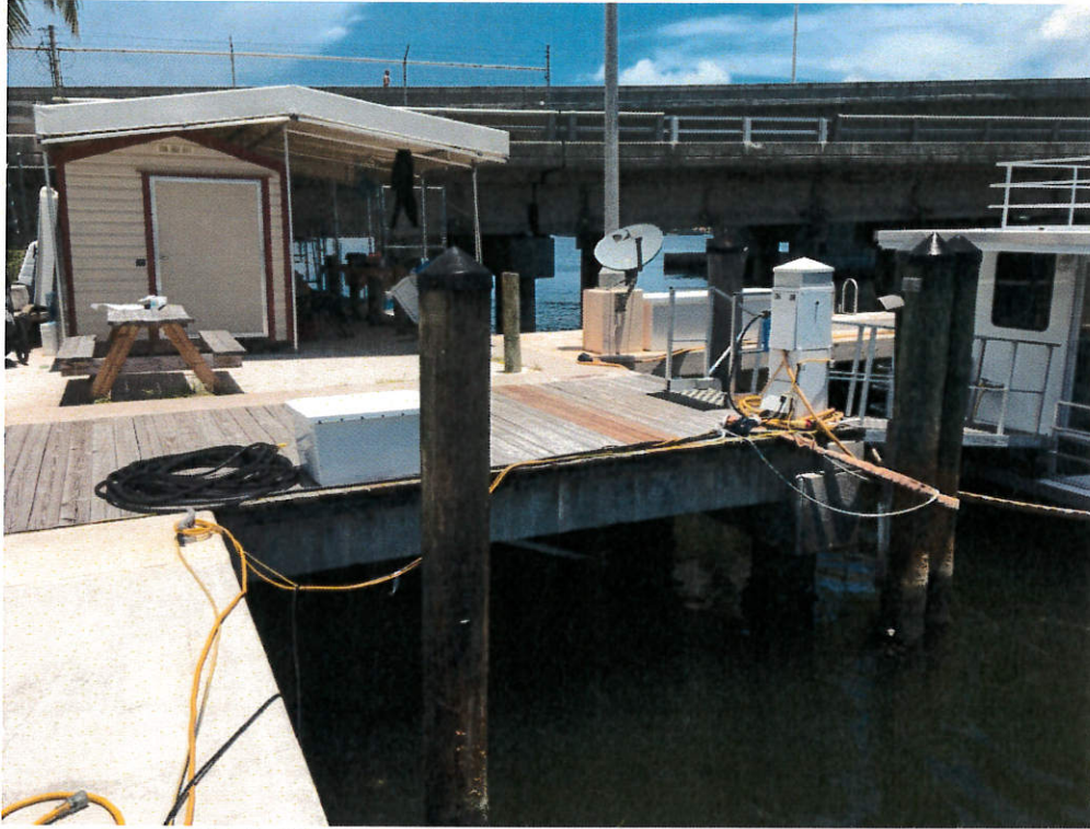
Photo 11: Transition from Pier 5 to Pier G (beyond).
