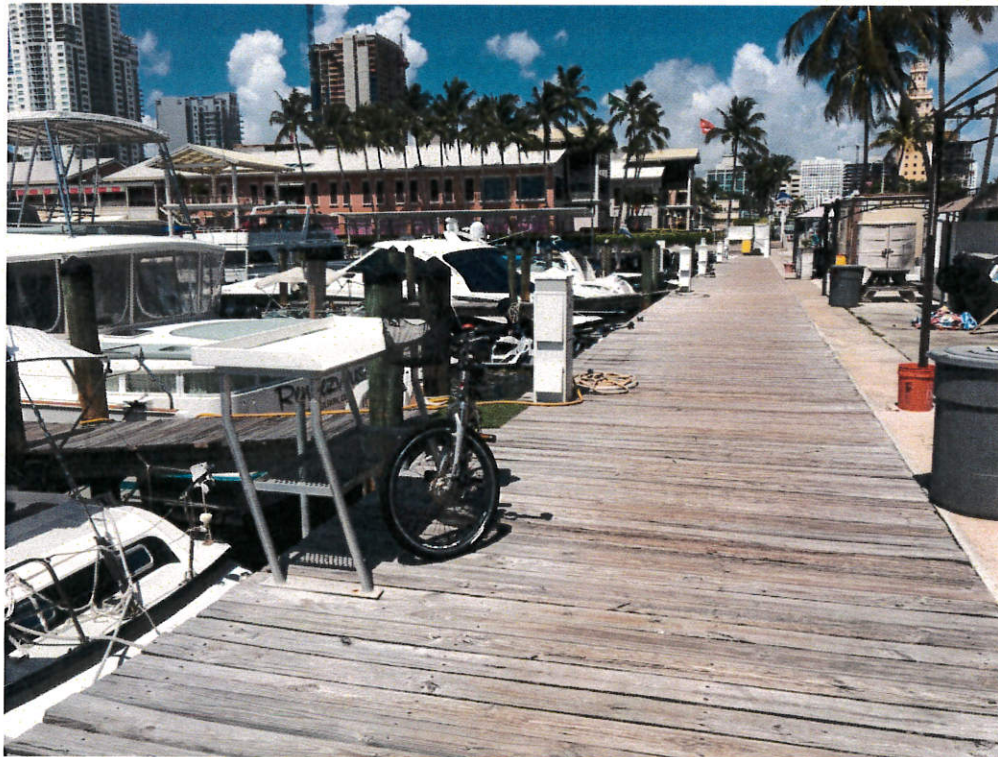
Photo 8: Existing bulkhead, pedestals, sidewalk and wood deck (looking west).
