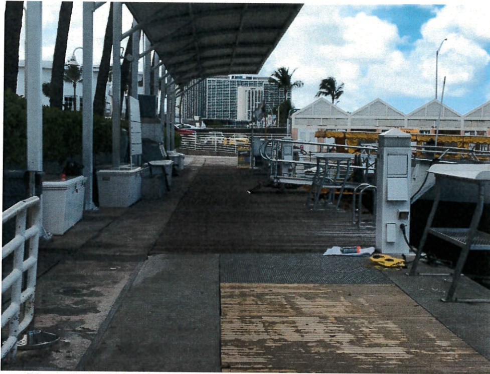
Photo 1: End of new construction with concrete beams (looking north)
