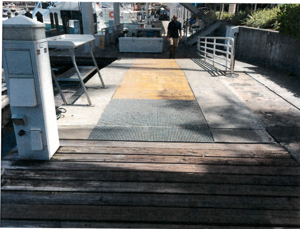
Photo 2: Beginning of wood decking construction (looking south).
