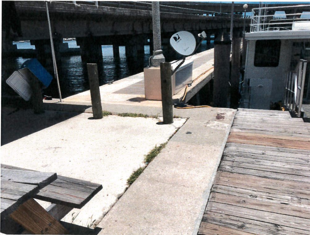
Photo 12: Transition from Pier 5 to Pier G (beyond).
