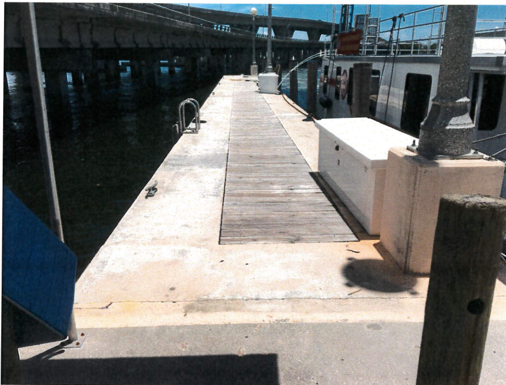
Photo 13: Overall view of Pier G (looking east).
