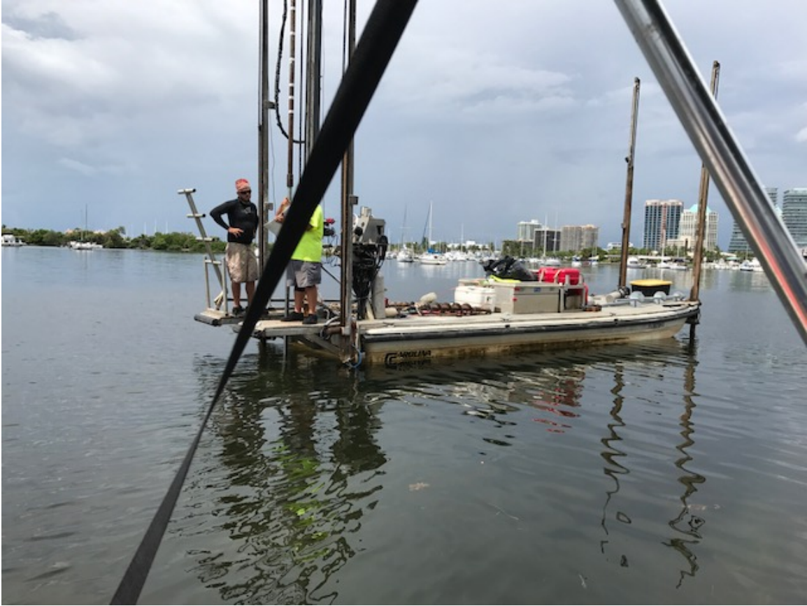
Figure A-2: Anchor installation barge at the Dinner Key Marina
