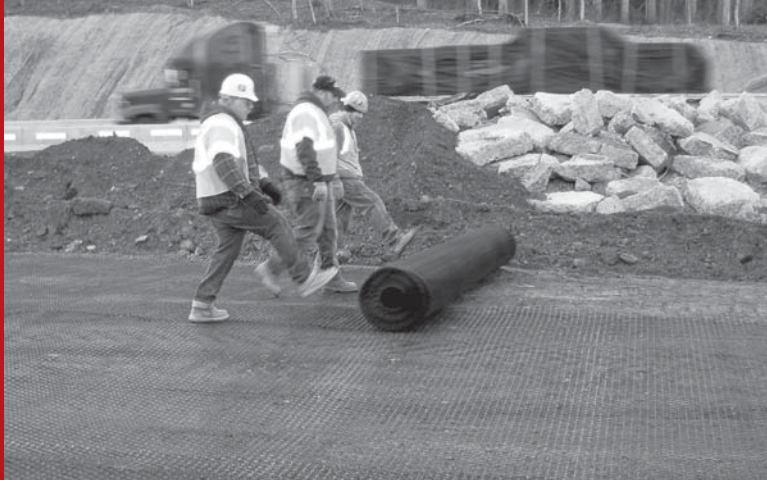
IMAGE 3: Rolling out Tensor® Geogrid.
