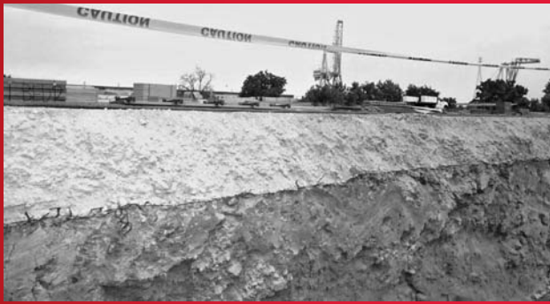
IMAGE 13: A backhoe excavation through Tensar Geogrid.
