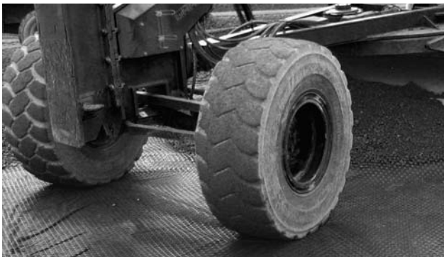
IMAGE 12: Geogrid can be trafficked directly by rubber-tired equipment.
