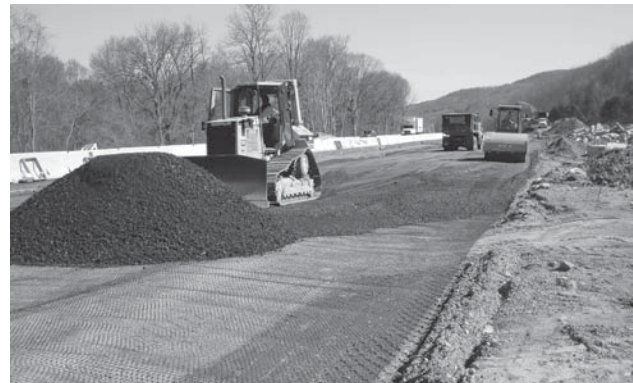
IMAGE 9B: Spreading aggregate fill over Tensor Geogrid.
