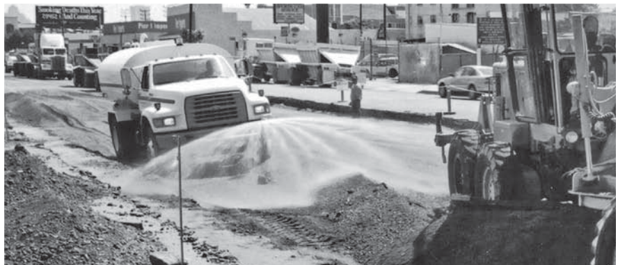
IMAGE 10: Moistening the fill before compaction.
