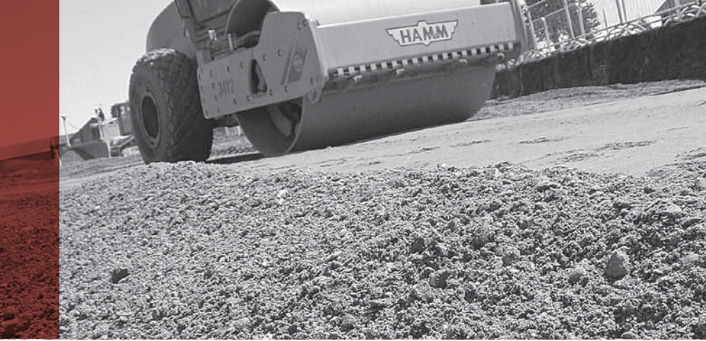
IMAGE 11: Compacting the aggregate fill.
