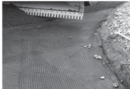
IMAGE 5: Placing Geogrid to accommodate curves.
