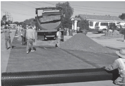
IMAGE 4: Geogrid should overlap in the direction of advancing fill.
