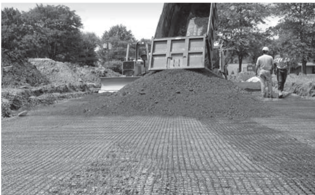
IMAGE 9A: End dumping aggregate fill on top of Tensor Geogrid over soft subgrade.
