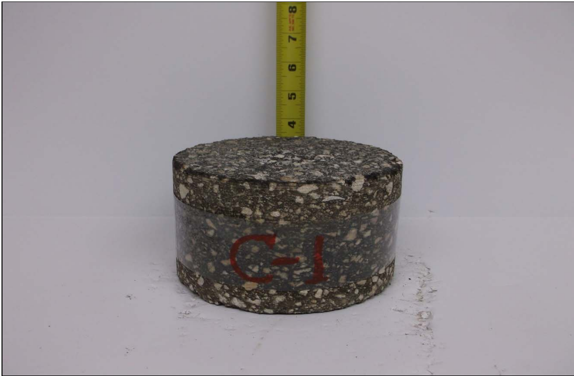
Asphalt Core No. C-1 Core Thickness 3.6 in.
