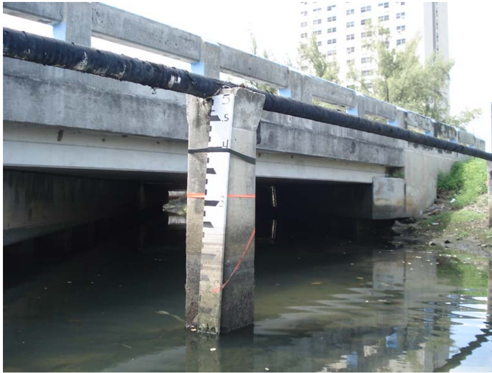
Stream gauge within Wagner Creek at the NW 14 th Avenue bridge.
