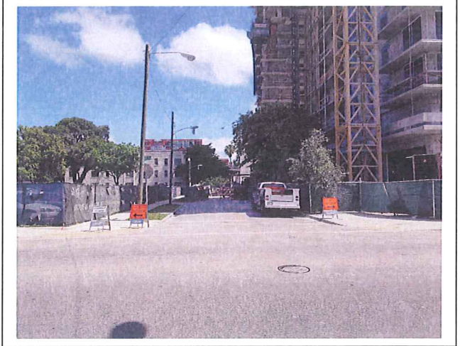
Photograph #6) Viewing North along NE Miami Ct
