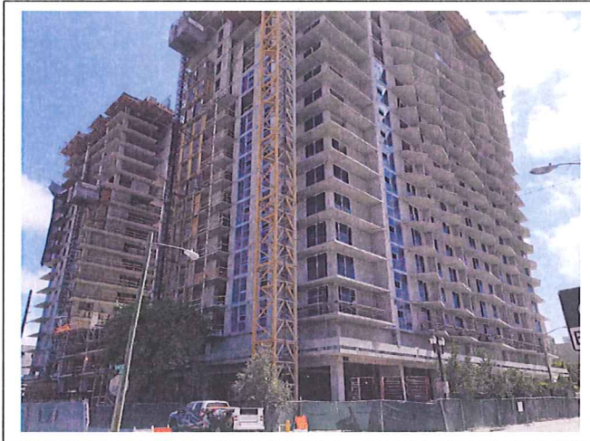
Photograph #5) Northeast neighboring building under construction
