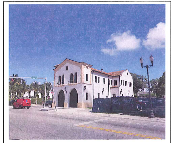
Photograph #8) Northwest neighboring office building
