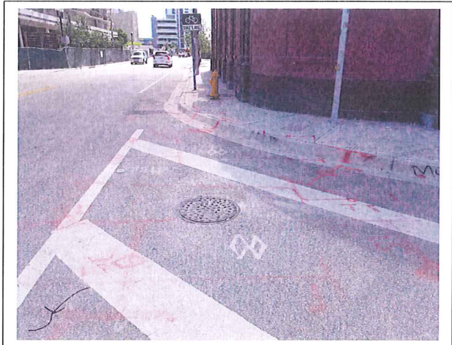
Photograph #18) Sewer manhole Northwest corner of subject site
