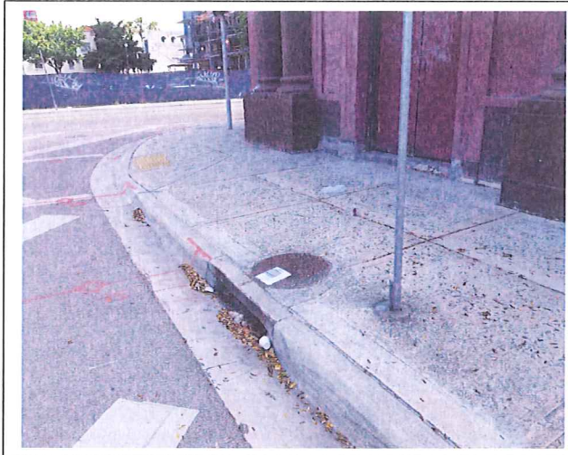
Photograph #17) Storm drain West of subject site
