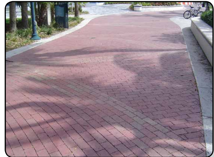
The image above shows pavers used along a riverwalk. All hardscape material shall conform to the transition zone requirements.
