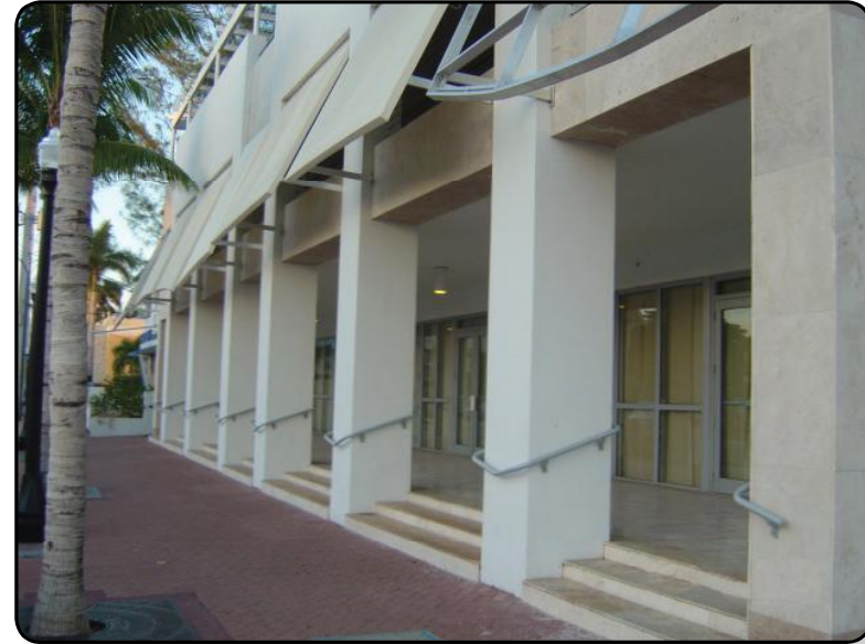
In cases where abrupt elevation changes are necessary, they should blend into the overall design of the facade as shown in the arcade above.
