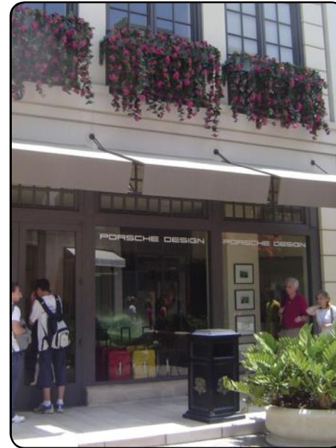
Highlighted entryway feature along the facade.
