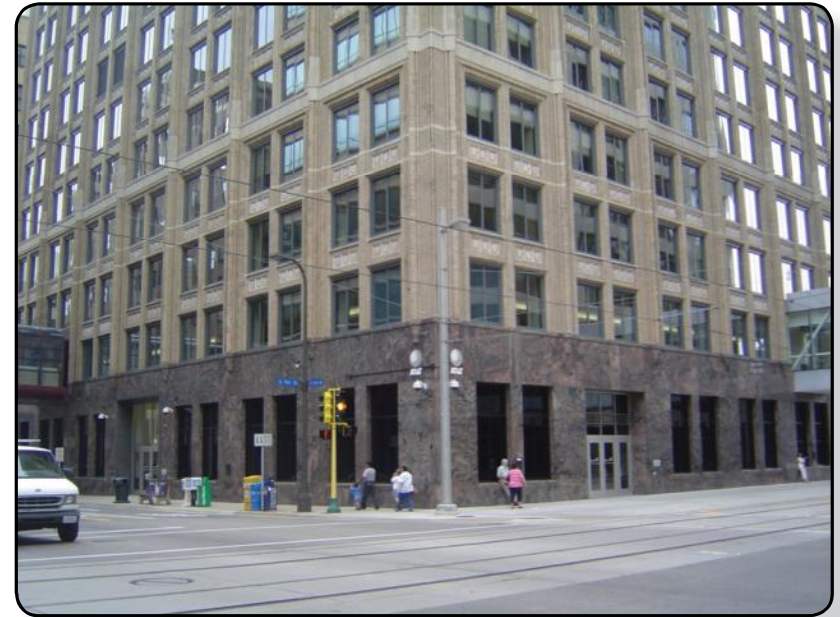
This building illustrates a good example of bringing the building facade down to the pedestrian scale, by a simple change in building materials and modifications to the facade plane.
